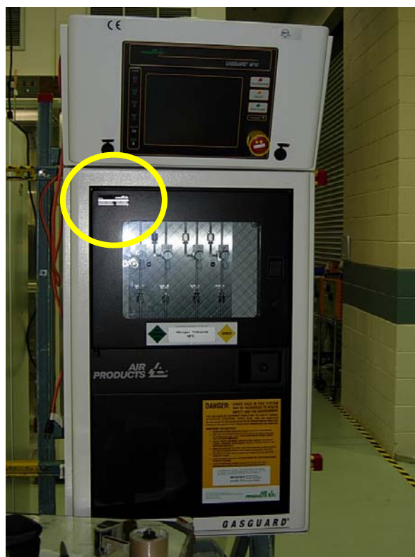
Figure 3: The AP10 Gas Cabinet equipment commodity code number (circled above) can be found on the enclosure door.
