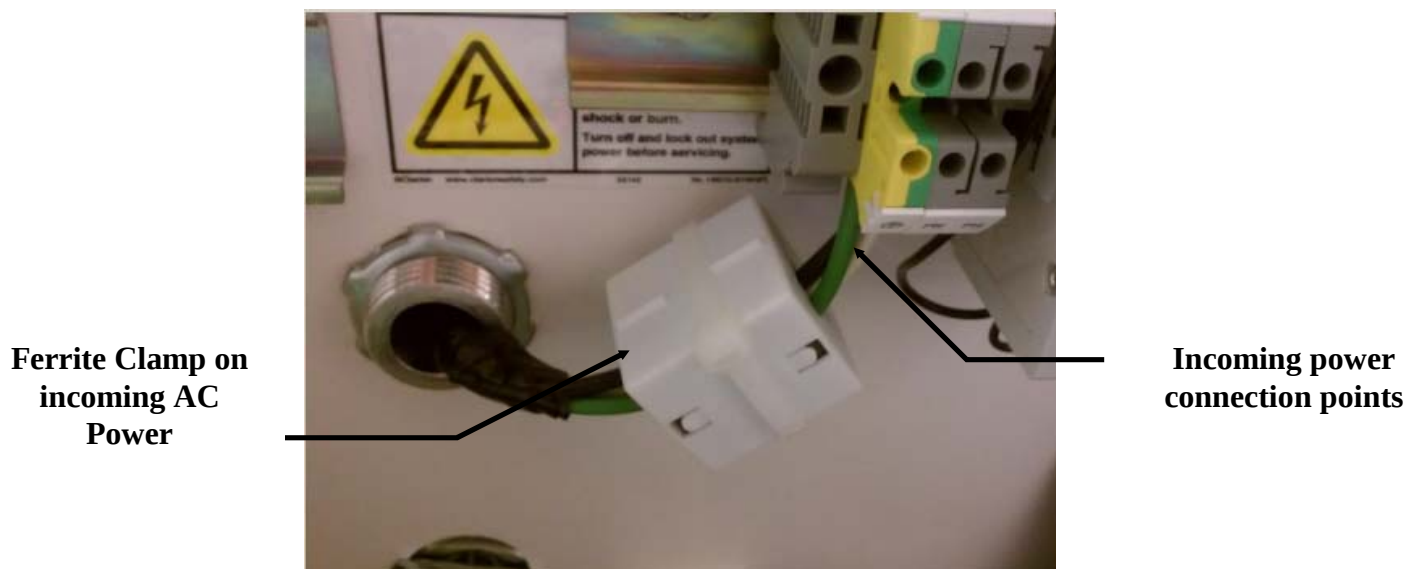
Figure 4.3: Inside View of GASGUARD APx Controller
