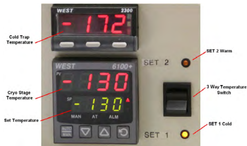
FIGURE 7-11 TEMPERATURE CONTROLLER DISPLAY
